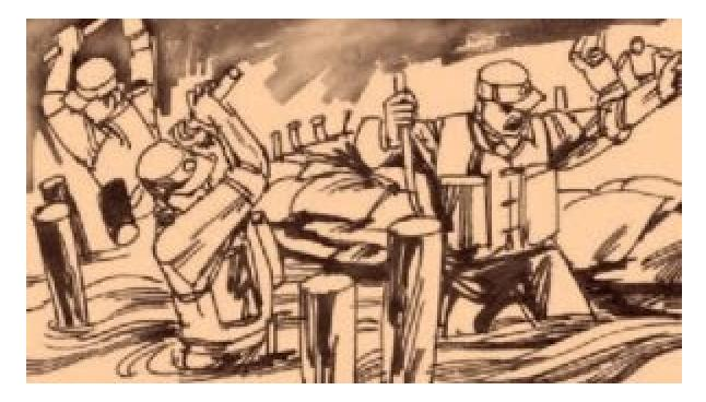
Later a 200-member special force group from Zhangjiakou, who were trained in levee repair came, and build pilings around the rupture. Afterward, they used pilings to stabilize the prefabricated panels, then, they poured in mud and rocks, eventually sealing the opening.
