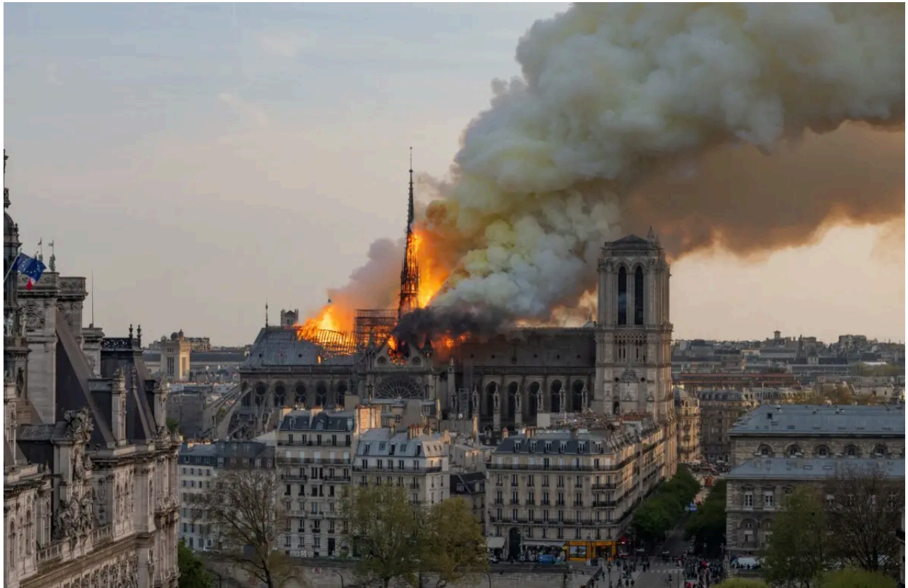
Smoke billows as flames burn through the roof of the Notre-Dame de Paris Cathedral in Paris on April 15, 2019. Fabien Barrau/AFP via Getty Images
